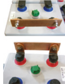
Fig. 5-18: Installing the end terminals (connection plates)
