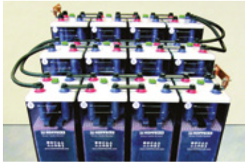
Fig. 5-16: Using row connectors and step connectors
