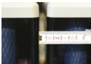
Fig. 5-13: 10 mm clearance between the batteries
